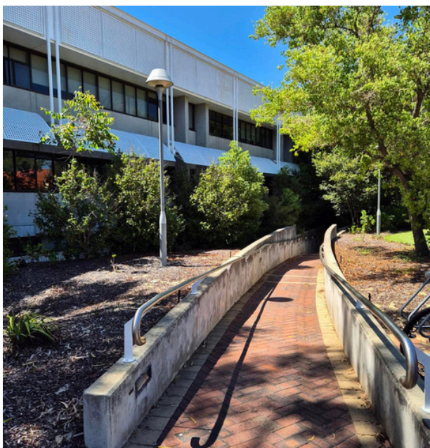
Accessible ramp to the building entrance
