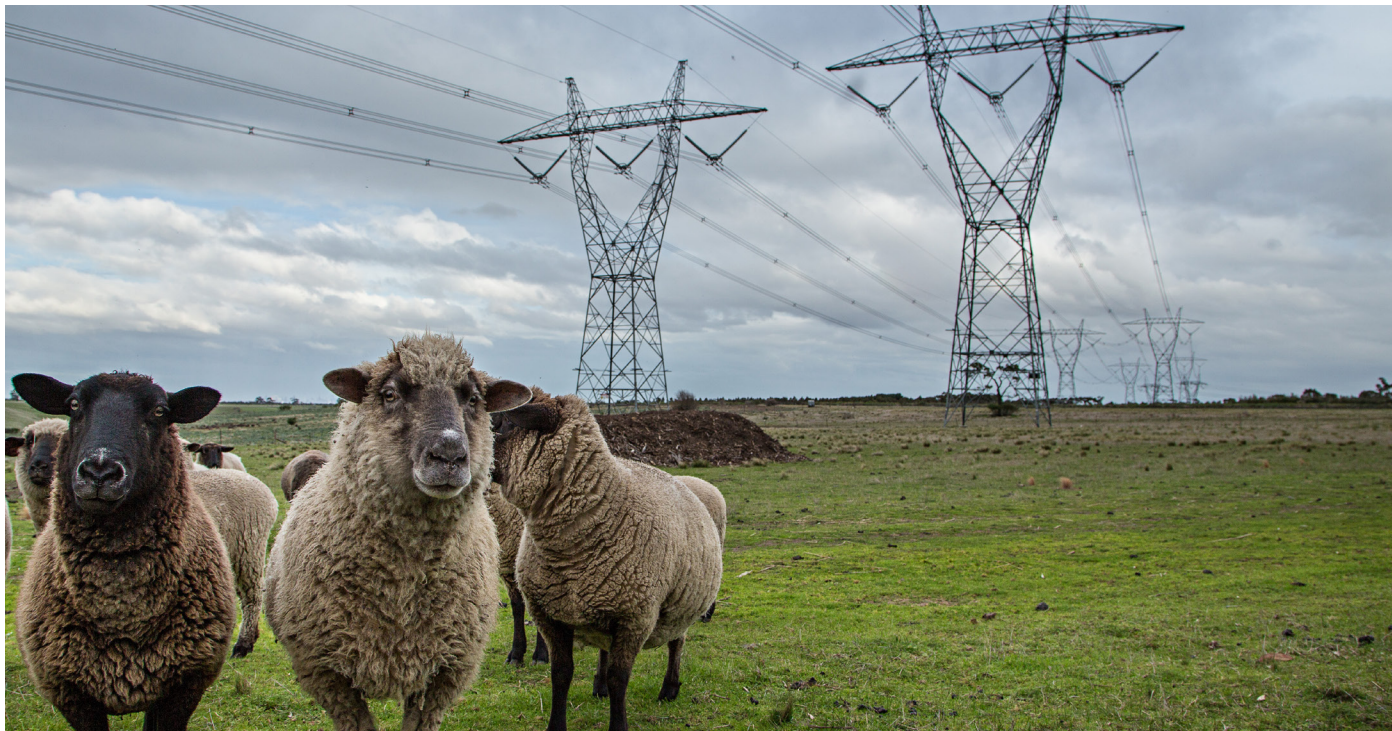
Image: High-voltage powerlines often run through rural areas, including farmland. Adobe Stock (n.d.).
