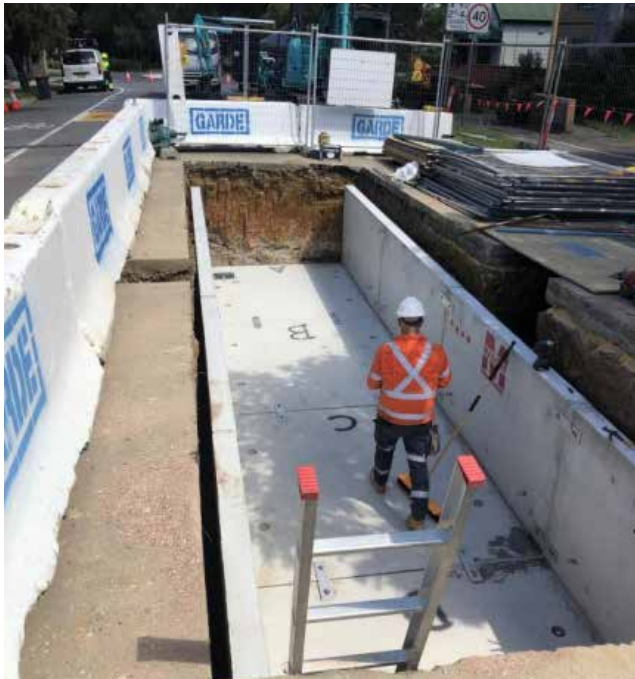
Figure 21. Powering Sydney’s Future—330kV Cable Joint Bay (Transgrid)
