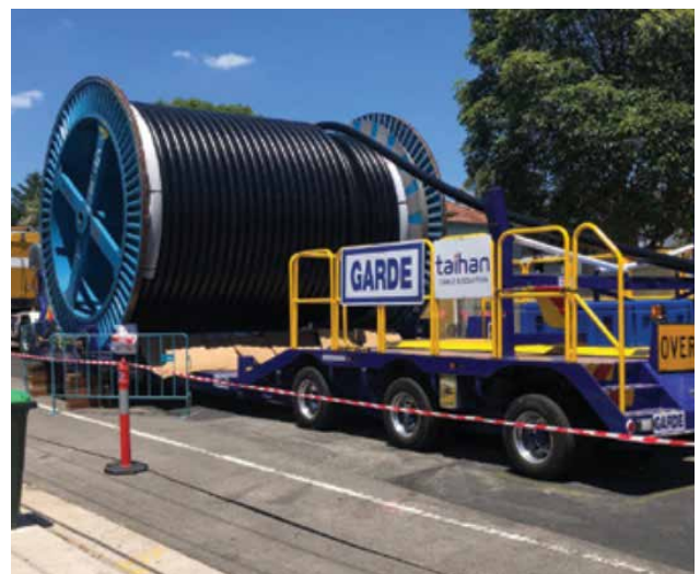
Figure 23. Powering Sydney’s Future—330kV Cable Drum (Transgrid)
