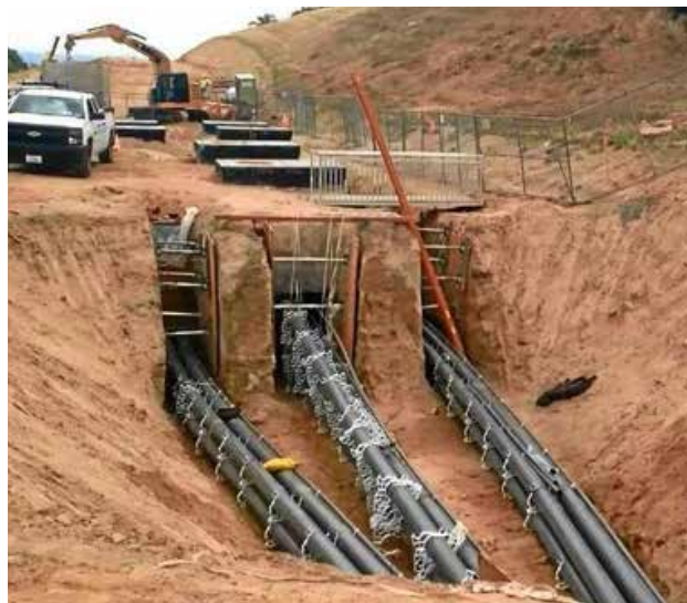
Figure 7. Tehachapi 500kV Underground Cable Installation (dailybulletin.com)
