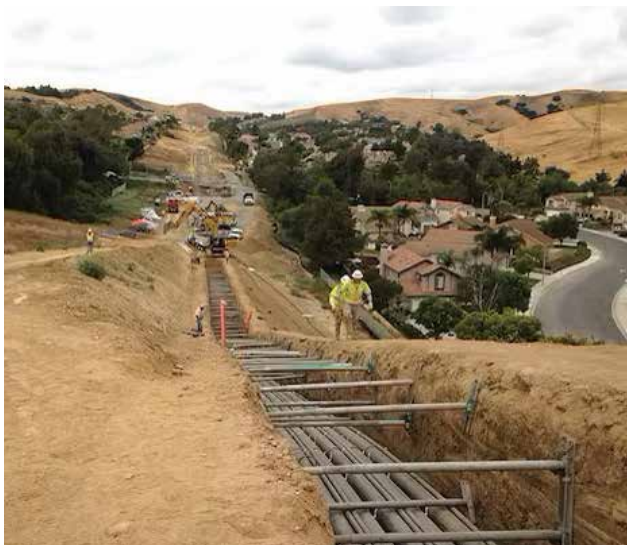
Figure 6. 500kV Underground Cable Trench Installation at Chino Hills (T&D World)
