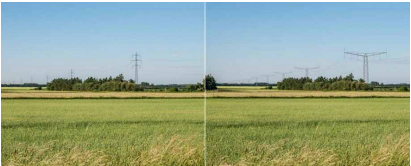
Figure 12. Existing 150kV OHTL (left) and Proposed 400kV Structures (right) (Energinet)
