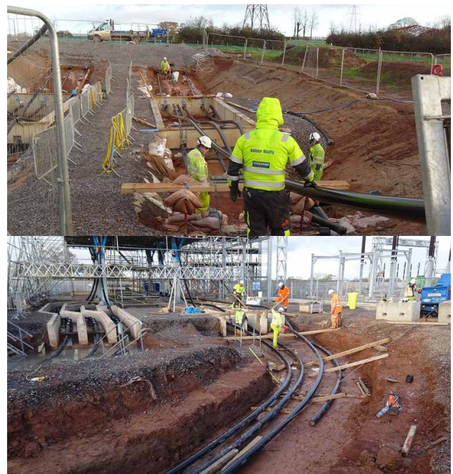
Figure 27. Hinkley Point C Connection Project--400kV Underground Cable Works (National Grid)
