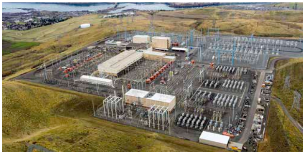
Figure 35. HVDC Converter Station (ABB 17 )
