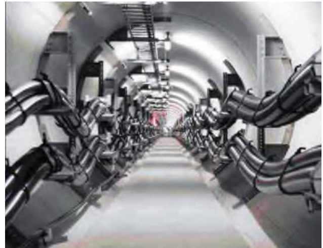
Figure 23. Cable Tunnel Installation (Nexans / CIGRE 2017 [12])
