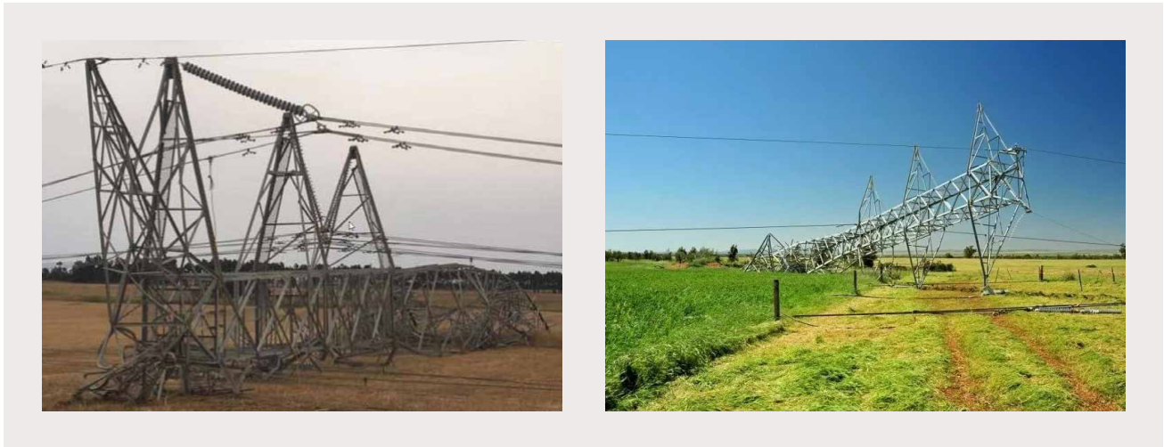
Figure 9. Fallen 500kV Double Circuit Tower, Victoria (Zinfra Pty Ltd.) and 275kV tower, South Australia (ABC News: Dean Faulkner)
