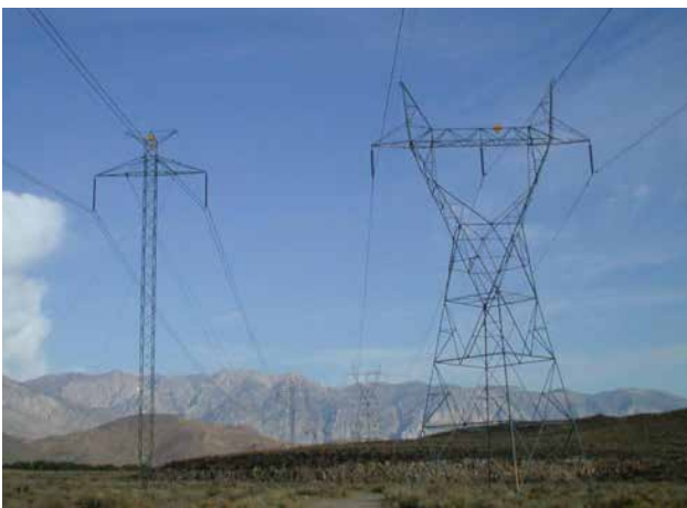
Figure 29. Single Circuit Guyed HVDC Overhead Transmission Line (Left) and Self-Supporting HVAC Transmission Line (Right) (AlternativeUniversity.net 16 )
