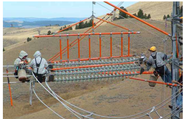
Figure 4. Live Insulator Change-out (North-western Energy UK)
