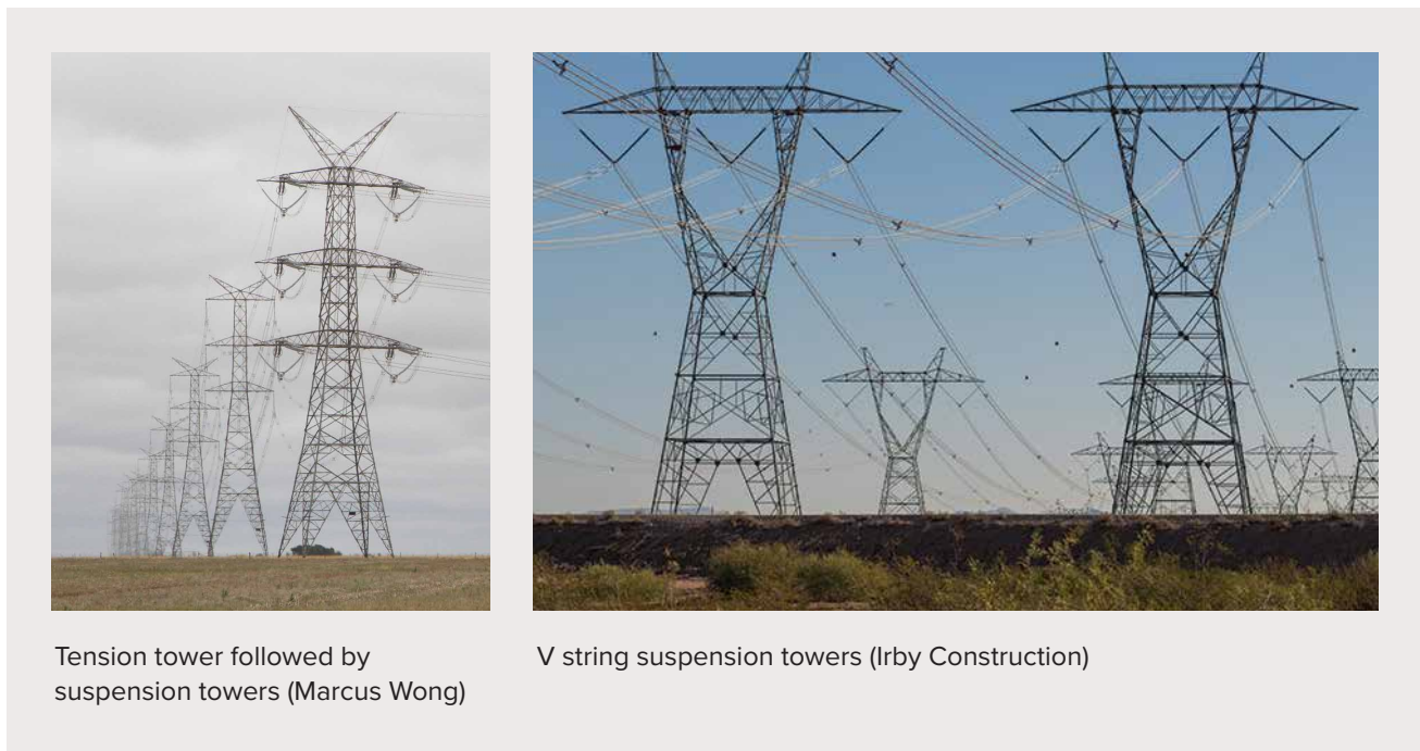
Figure 3. 500kV Double and Single Circuit Overhead Lines
