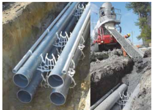
Figure 27 2x2 duct bank (left) and concrete backfill installation (right) [31]
