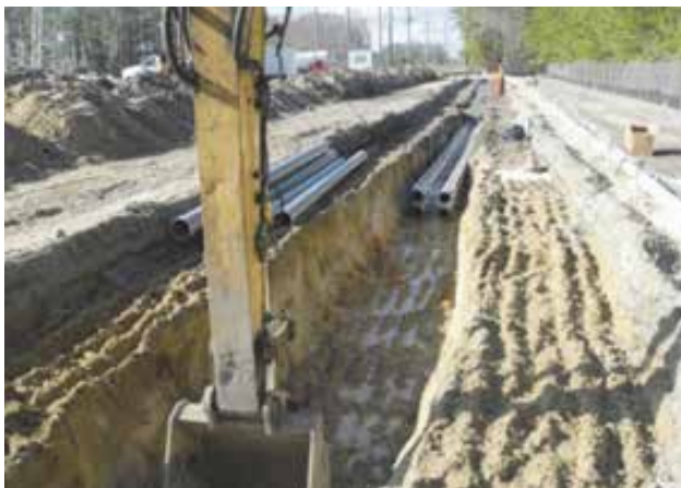
Figure 25 open cut excavation for cable system [31]
