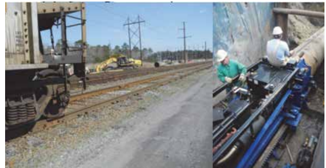
Figure 29 Pipe-jacking operation under rail sidings [31]
